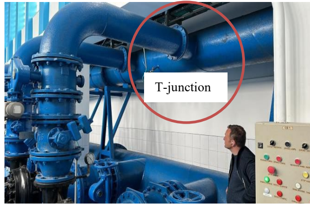
Figure 1. Discharge pipe and main collector – pumping station RAJA, Constanta
