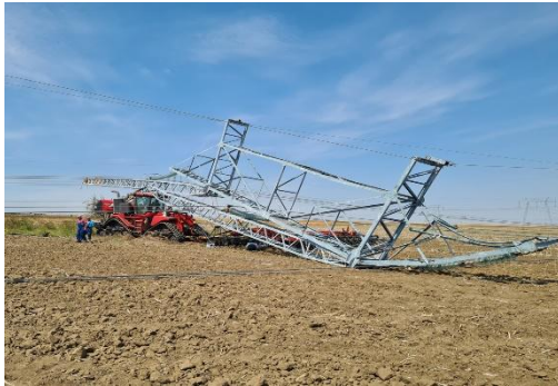
Fig. 4 Failure caused by damage of the transmission tower B174 on the 400kV Rahman-Dobruja line, 2021
