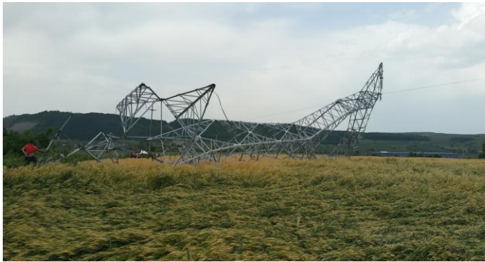
Fig. 1 Failure caused by tornado combine with strong wind gusts affecting the 400 kV Iernut-Gădălin power line and the 220 kV Iernut-Baia Mare 3 power line in June 2016
