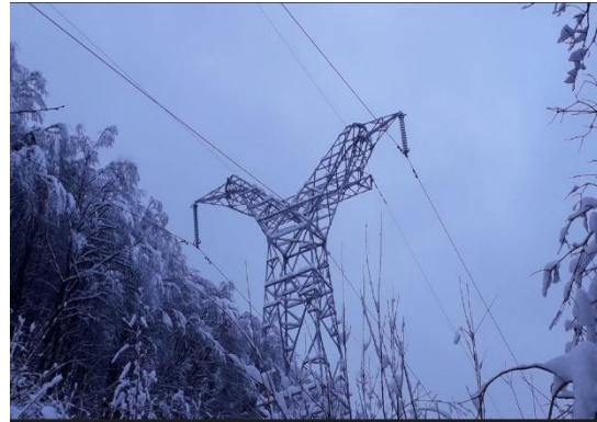
Fig. 3 Failure due to an ice storm on the 220kV Stejaru-Gheorgheni, 2016
