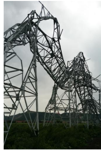
Fig. 1 Failure caused by tornado combine with strong wind gusts affecting the 400 kV Iernut-Gădălin power line and the 220 kV Iernut-Baia Mare 3 power line in June 2016
