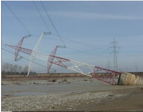
Fig. 2 Failure by flooding of tower B224 on 220kV Brazi-Fundeni line, 2008 [23]
