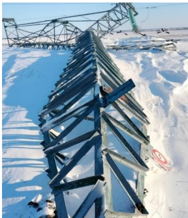
Fig. 6 Failure due to the aging anchoring system of transmission guided tower B189 on the 400kV Tariverde - Tulcea Vest line, 2023
