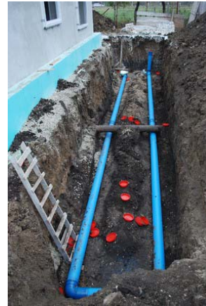
Fig. 3. Installation of the main side of EAHX tube
