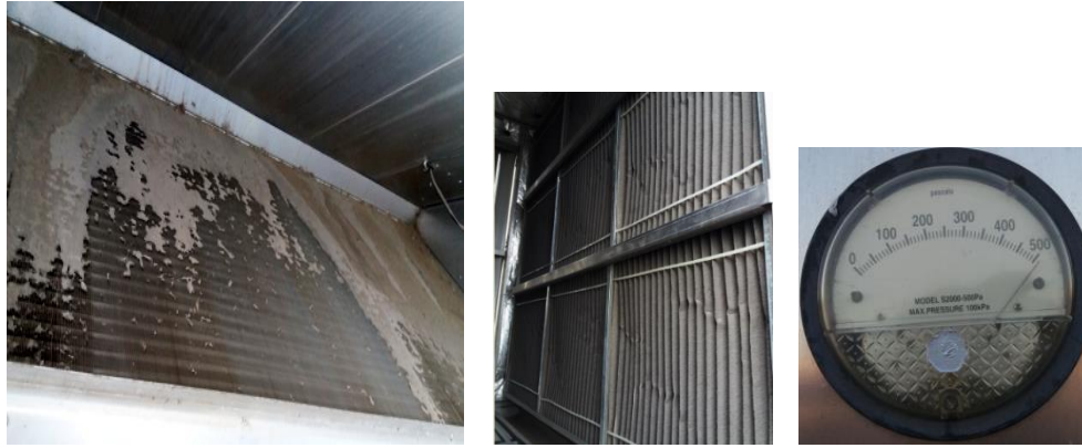
Fig. 2 Condenser coil and filters under fouled conditions
