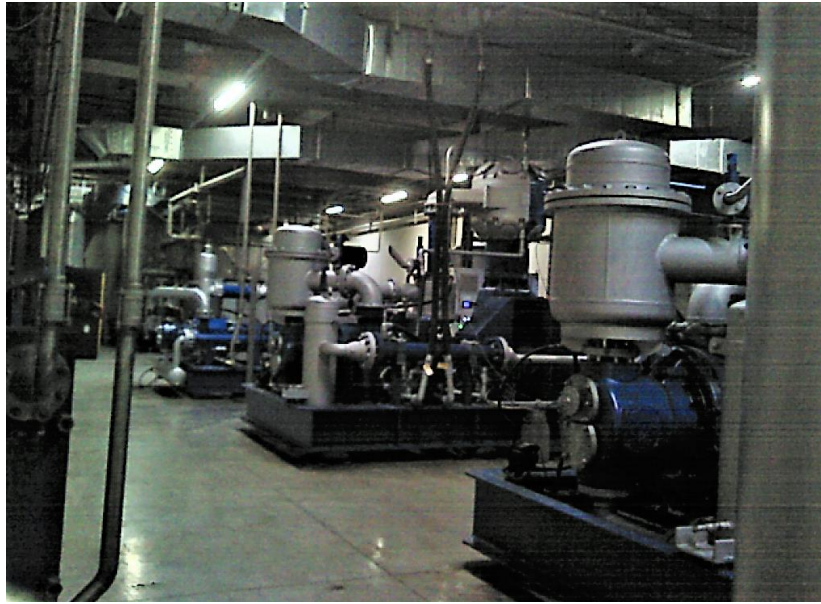
Fig. 2 The compressors station of PET bottles plant (Author's image).
