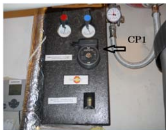
Fig 3: General view of the circulation pump (CP1) placed on the circuit solar vacuum collectors - double coils of the two storage tanks
