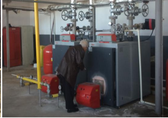
Fig. 3. The gas fired hot water boilers from DTP no. 2.
