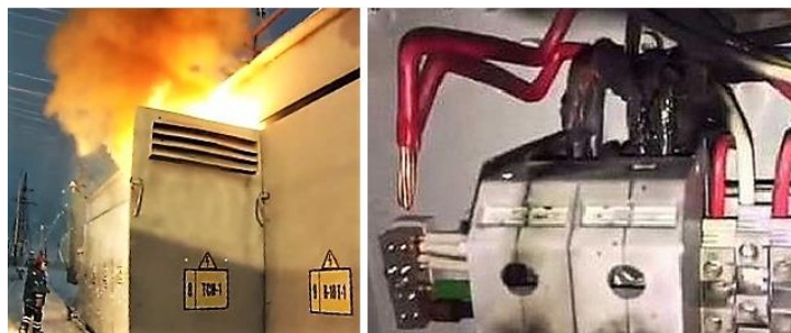
Fig. 2 Fires at electrical boards
