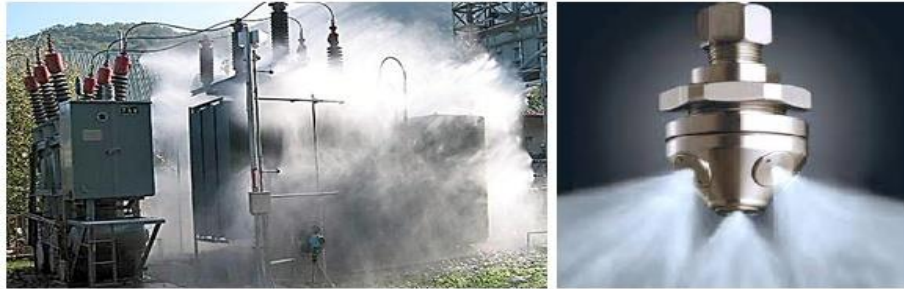
Fig. 9 Fixed water mist extinguishing system in acting and a spray nozzle.
