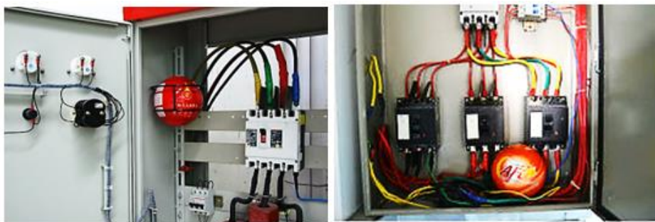
Fig.12 Fixed dry powder extinguish system
