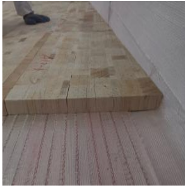
Fig 8. No clearance left in layering
