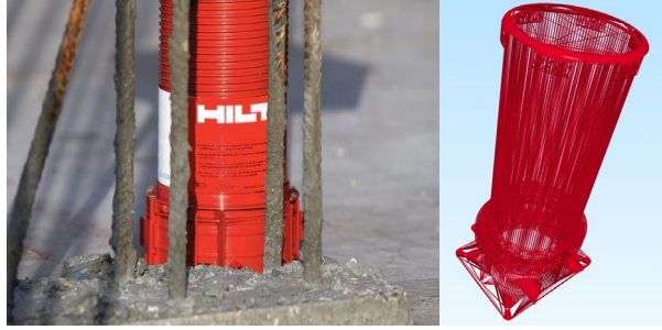
Fig. 9. Real-World Implementation and AR-Enabled Visualization of a One-Step Firestop Cast-In Solution
