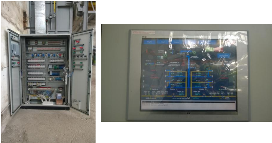
Fig. 3. Automation PLC cabinet and HMI panel [19]
