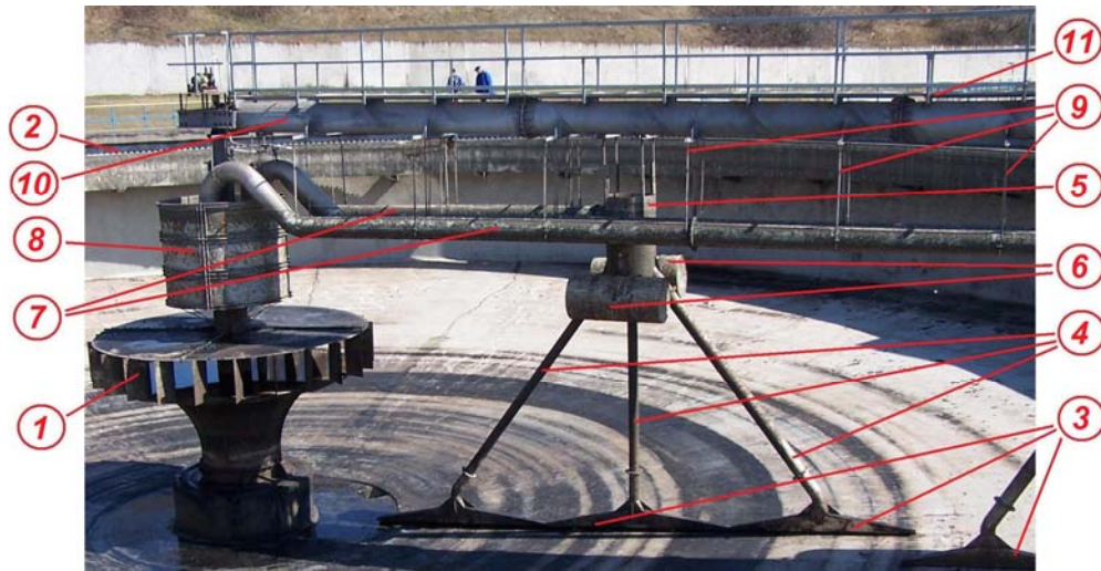
Fig. 1. Components of a circular settling tank and the rotating bridge
