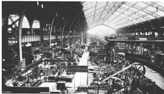
Fig. 6. Ferdinand Dutert, Victor Contamin, Machines gallery, Universal Exposition in Paris, 1898. The hall had a bay with only one opening of 115m × 420 m.
