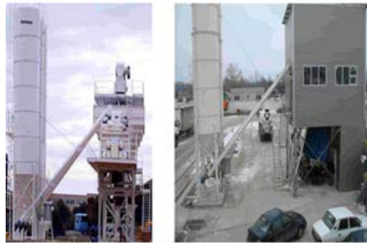
Fig. 6. Concrete station before and after building the enclosure
