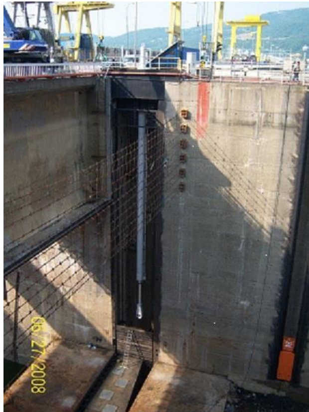
Fig. 2. Hydraulic servomotor of the intermediate gate of a lock (IRON GATES I Hydropower and Navigation System)
