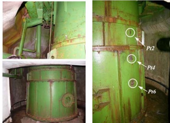
Fig. 2. The Francis turbine draft tube cone with air injection system (left) and the pressure taps installed on the cone (right).
