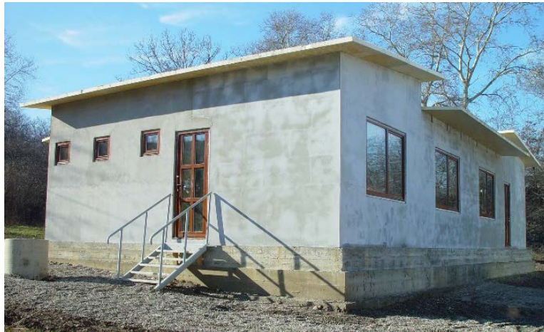
Fig. 4. House from composite panels only, designed as kindergarten
