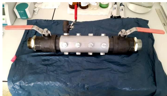
Fig. 2. The collector containing biofilm, the injection water and corrosion products
