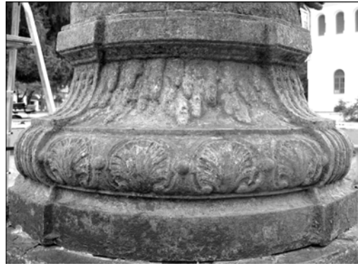
Fig.3. Detailed view of the metal base
